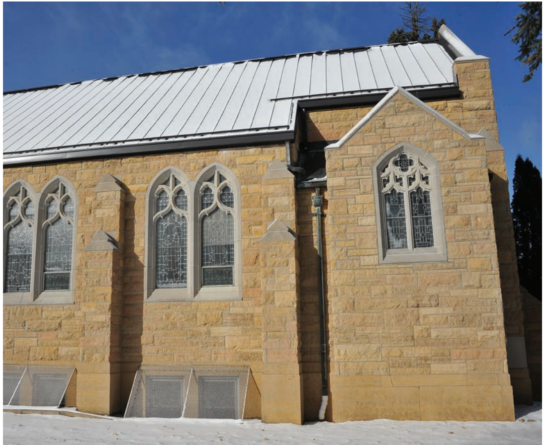
Cleaned and sealed sandstone complete!
