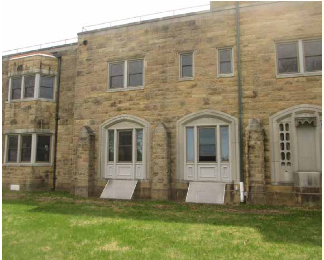
Building Sandstone Discoloration.
